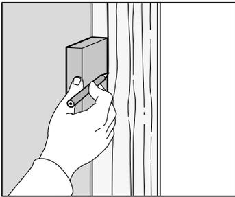
If the wall isn't level and flat, the filler piece must be cut to fit to the wall's shape. To do this, you'll need a filler piece, measuring tape, small block of wood about 2.5-3.5 cm thick and pencil.
